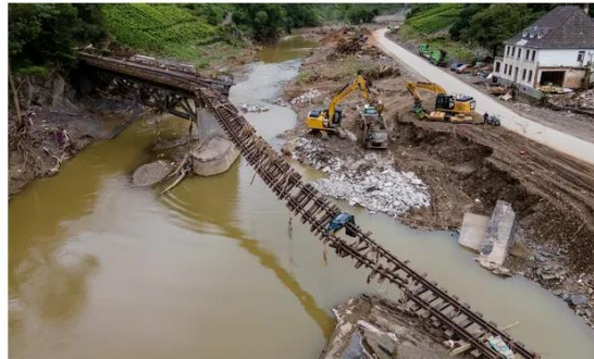
■ A damaged railway bridge five weeks after the flooding of the River Ahr in Rech in the Ahrweiler district of Germany on 19 August. Photograph: Friedemann Vogel/EPA
